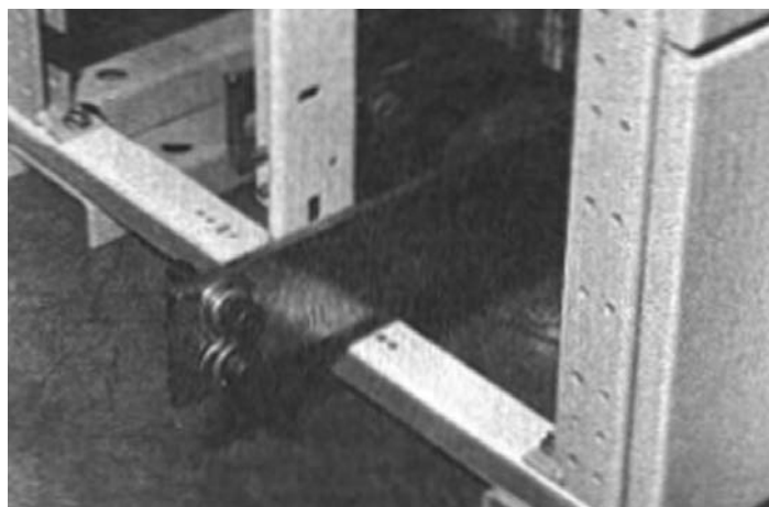
Figure 14. Splice Plate Attached to Freedom FlashGard Neutral Bus
