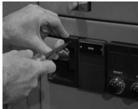
Figure 35. Defeater Mechanism
