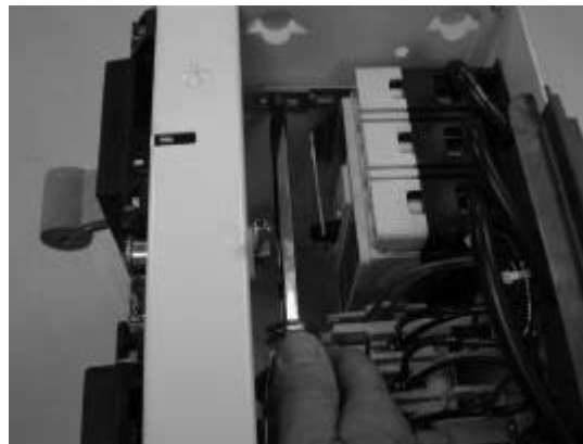
Figure 32. Operating Handle Linkage Adjustment
