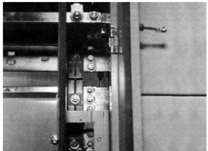
Figure 5. Access to Left-Hand Splice Plate Connections
