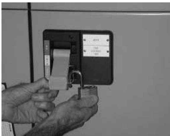
Figure 36. Locking Out a Disconnect
