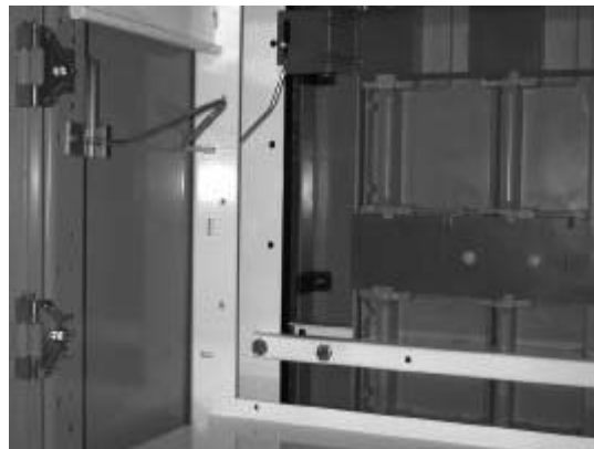
Figure 33. Shutter Arm Linkage
